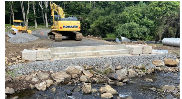
Foundation for temporary bridge
