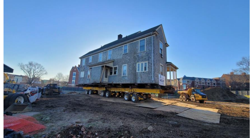
4 Gilbert Road House Relocation
