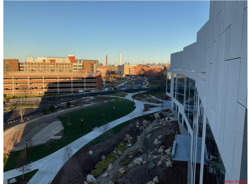
North Elevation Looking East
